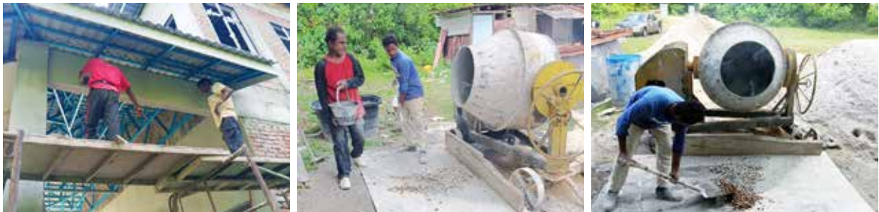
HCIB contributed Yellow Panda cement bags to support the development of KBBT's multi-purpose community facility.
